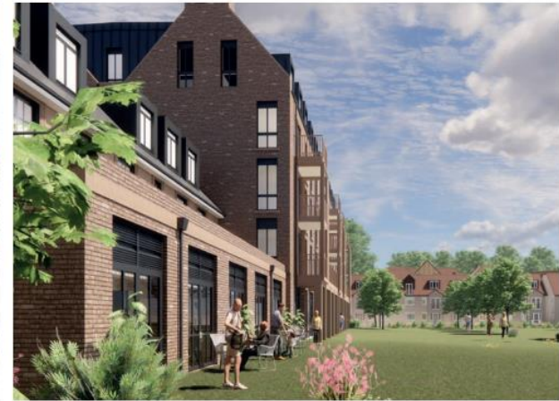
2. View from the front of Alexander hall, looking towards southern extension of block A
